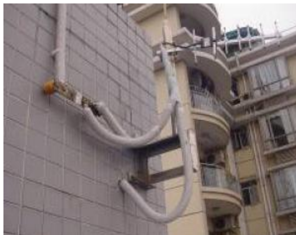
Cable layout through walls – “U” Dripping bend
